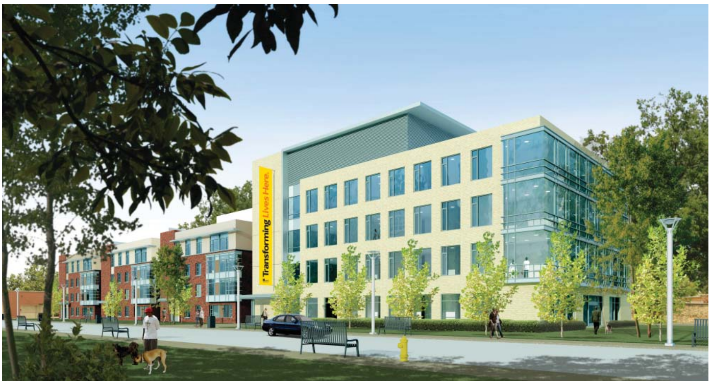
CAMH Redevelopment, Phase 1A, C3
