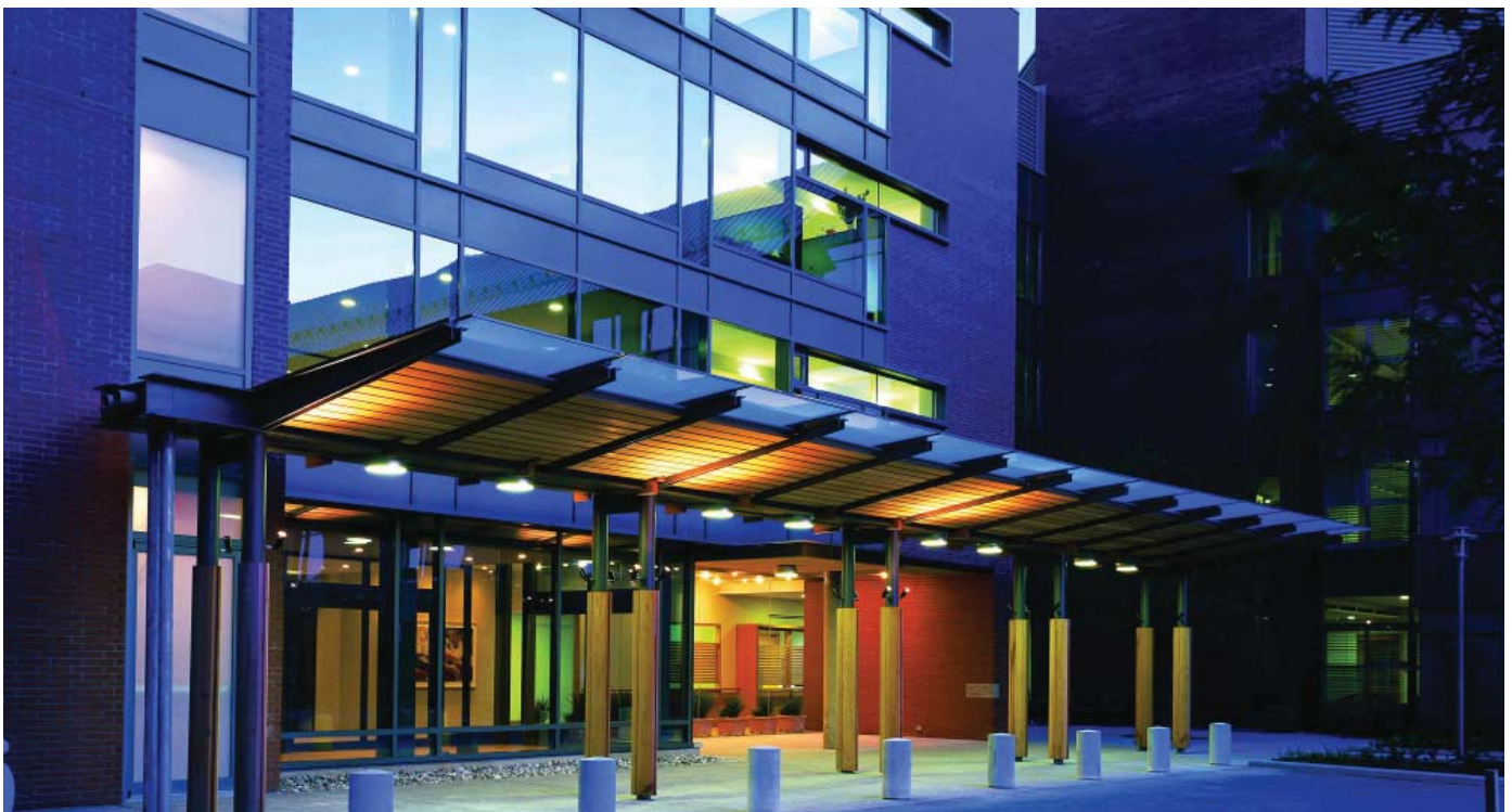
Providence Centre, Toronto, Montgomery Sisam Architects | Kuwabara Payne McKenna Blumberg Architects
