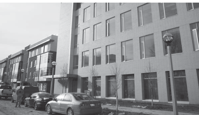
The first four buildings of Transforming Lives Here, the CAMH redevelopment project, are nearly complete and will open in April 2008. The buildings feature ample natural light, a decidedly non-institutional look, and outdoor courtyards. This is the first step in the redevelopment of the 27-acre Queen Street site into a mixed-use urban village, where CAMH's new facilities will sit side-by-side with new shops, cafes, residences and offices.
